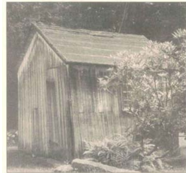
Shown is a farm outbuilding on the property of the William Noyes house.
