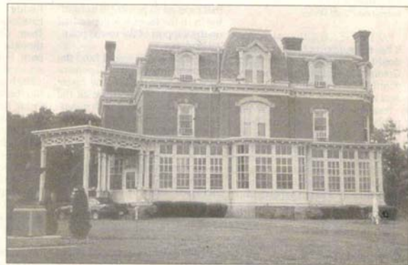
Above, the John Carter Brown Estate today is best known as Scalabrini Villa. Below is the property's carriage house.
